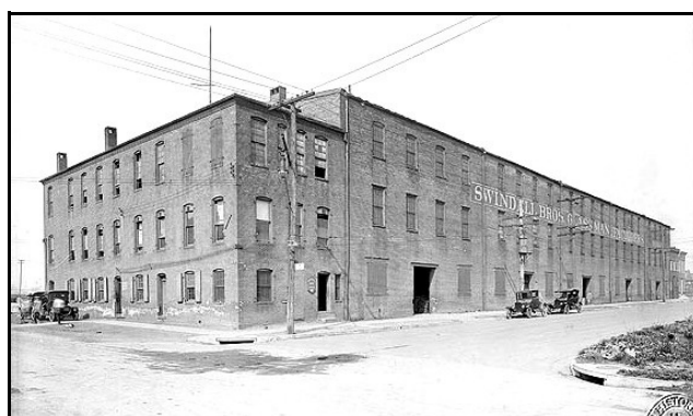
Figure 4 – Swindell factory (Maryland Historical Society)
