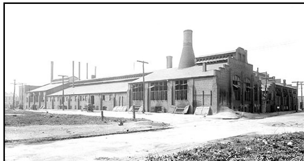
Figure 3 – Swindell factory (Maryland Historical Society)
